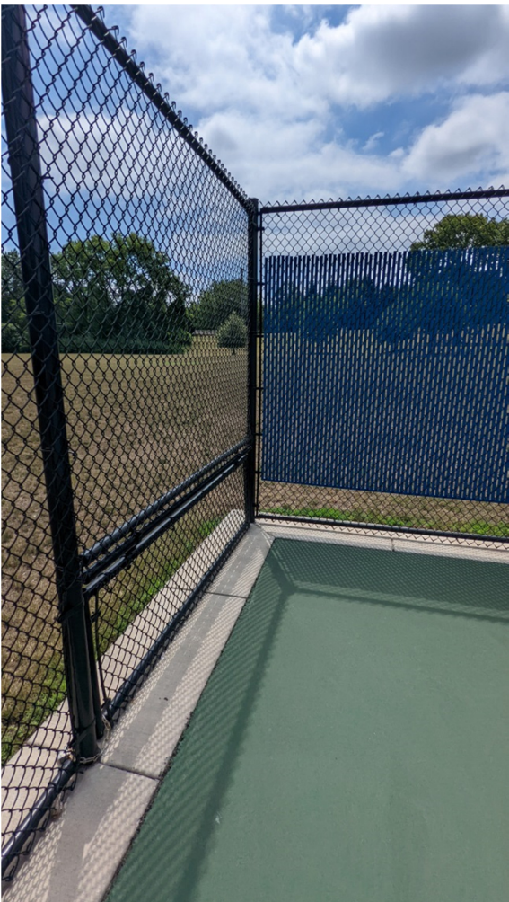
Photo 5, Concrete Fence Footings
