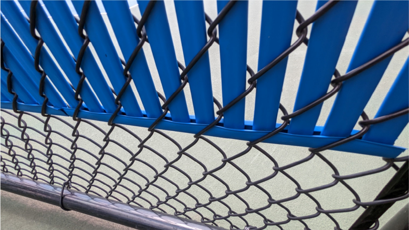
Photo 7, Windscreen Fence Insert Details
